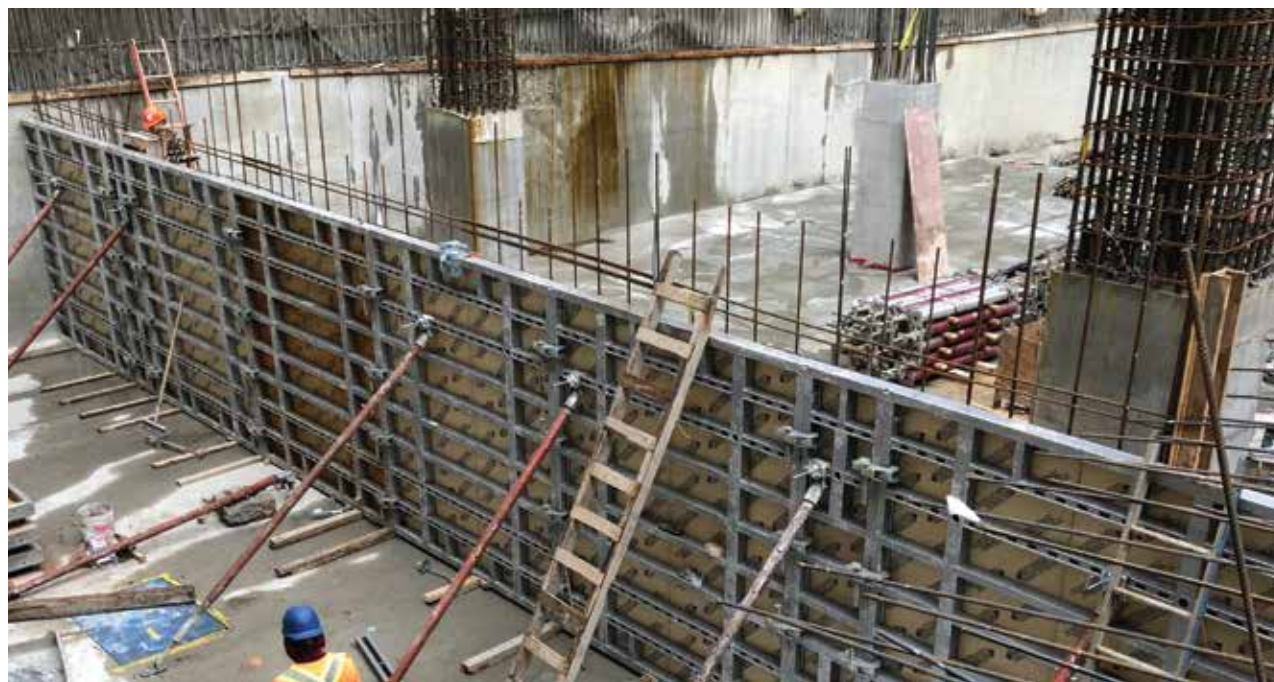
Large PROMAX Panel assembly fly in position with crane
