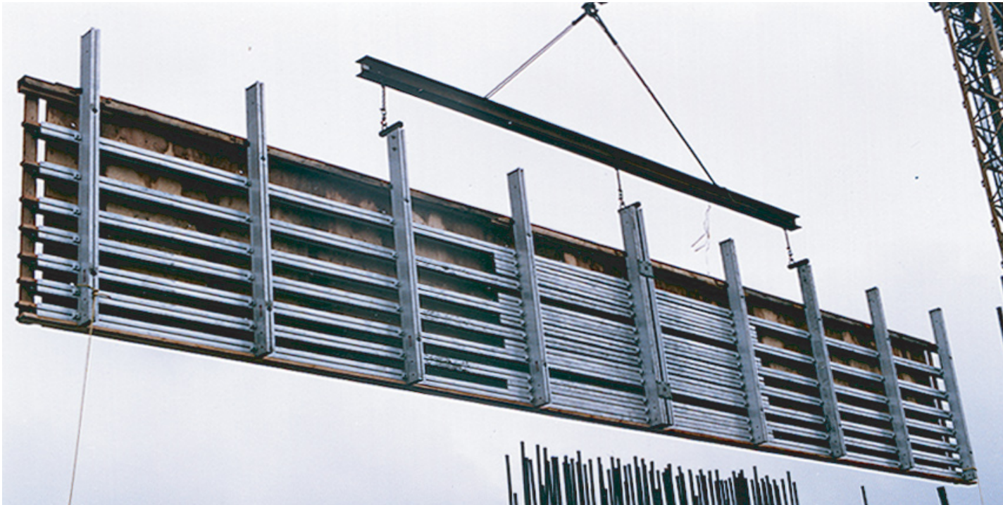
Gang Form Panel 10 ft high x 56 ft long has WH-750 Strongbacks at 7'-0" apart with only two taper ties per strongback.
