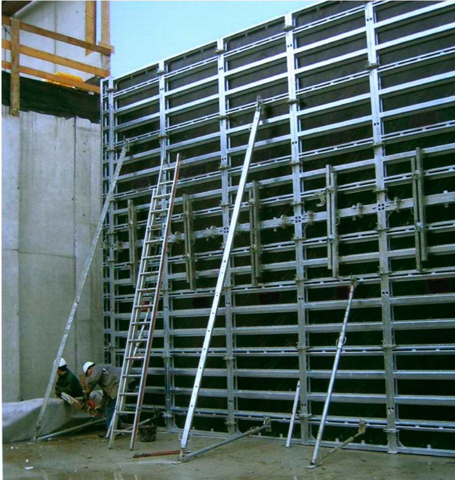
Large and high wall areas formed with two staked STERLING Panels 2.70 m high for single concrete pour of 5.40 m.
