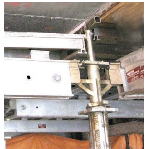
Drop Head lowered for 18 cm for dismantling of MODUDECK Beams and Panels, while at the same time it supports a newly poured concrete slab as re-shoring.
