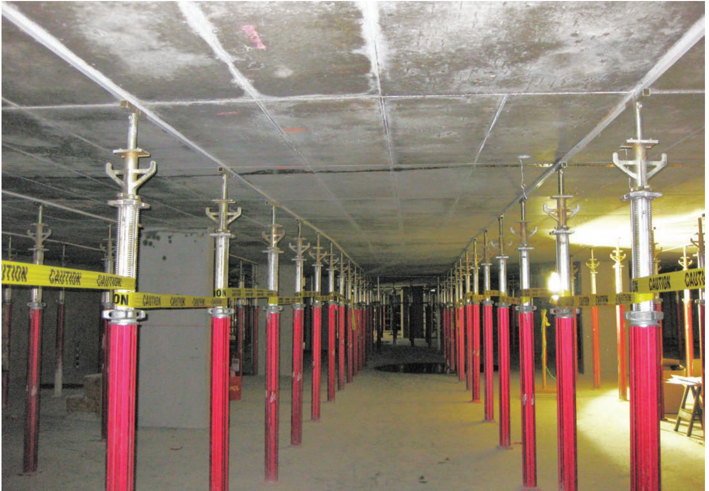
MEGA Shores with Drop Heads and cover strips stay in place as re-shoring after dismantling of MODUDECK Panels and MODUDECK Beams.
