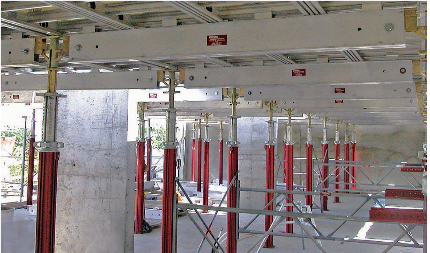
Lateral bracing frames between MEGA Shores.
