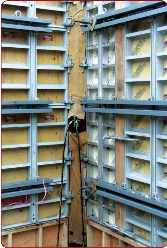
HYDRAULIC STRIPPING CORNER CONNECTING TWO PERPENDICULAR ALPAN WALLFORM PANELS.
