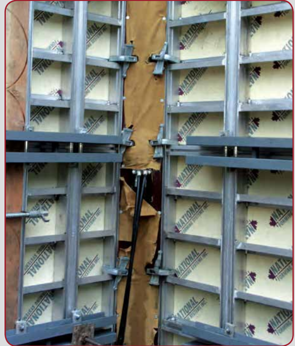
HYDRAULIC STRIPPING CORNERS CONNECTING PERPENDICULAR STERLING WALLFORM PANELS.
